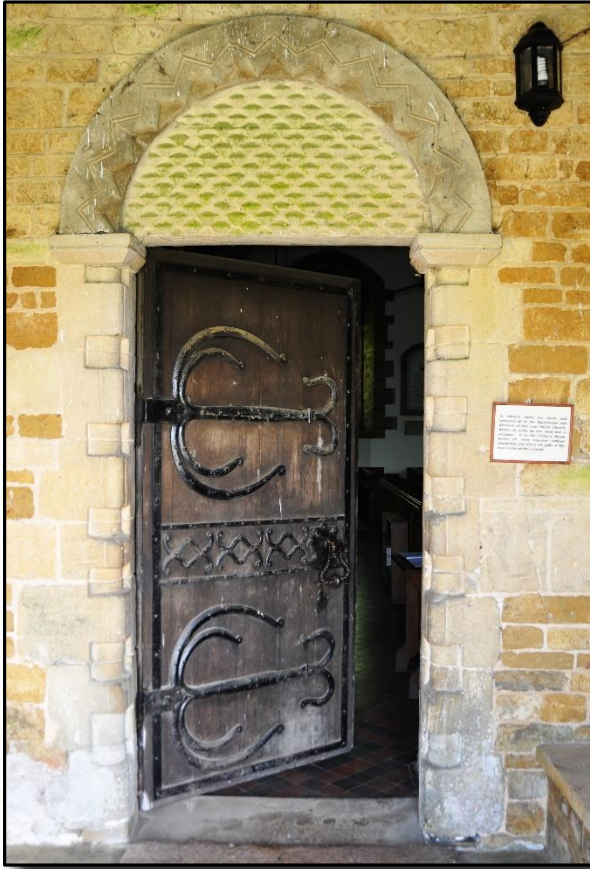
Inside the south porch the C12 Romanesque south doorway has alternating small and large edge-roll mouldings and a C12 fish-scale tympanum. (The zigzag-decorated arch is C19).
