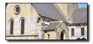
The western aspect reveals a variety of different window styles - the round-headed Norman style of the nave (not forgetting the round window in the west gable) and the flatter-headed, more Perpendicular style in the west wall of the south transept and south wall of the chancel.
