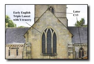
The basic structure dates from c.1180. The eastern windows are Lancet in style as seen in the pictures above. The name comes from their being shaped like the two-edged surgical knife formerly used to release blood.
