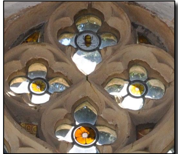
At the top of the windows in the south aisle can be seen several panels which are devoted to bumble bees and flowers which were one of the passions of the bee-keeping Revd Henry John Coleman who was rector from 1873 to 1907.
