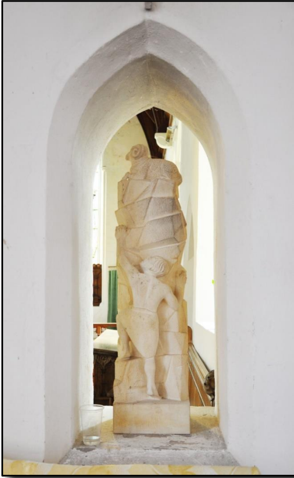
On each side of the chancel arch there is a squint for visual communication between the chancel and the nave.
