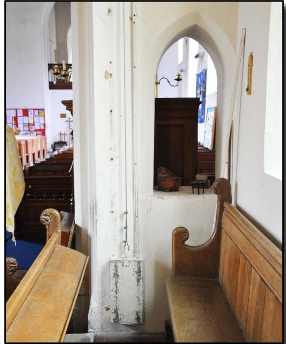
The chandelier is counter-balanced by a massive weight which allows for easy-lowering in order to light the candles . . . and to clean the brass!
