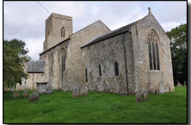
The window at the east end is a later replacement.
