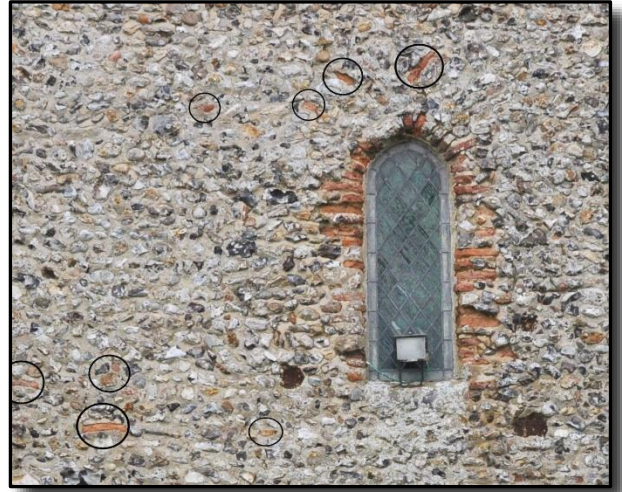
Low in the tower's west wall is a peculiar little round-headed (with just the suggestion of a point) window set into (perhaps Roman?) tiles. A few similar tiles perforate the rest of the wall as shown ringed above.
