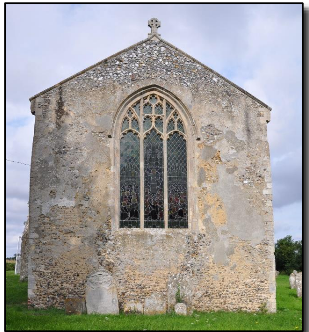
The tracery, although still of the Perpendicular style, is of a different pattern to the nave windows.
