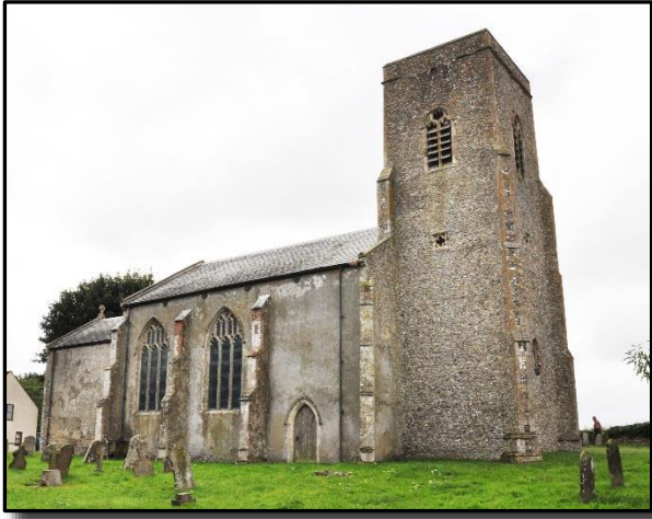
The church is said to date from late C12, C13 and C15 with C19 restoration. It is constructed of partially rendered flint with ashlar dressings.
