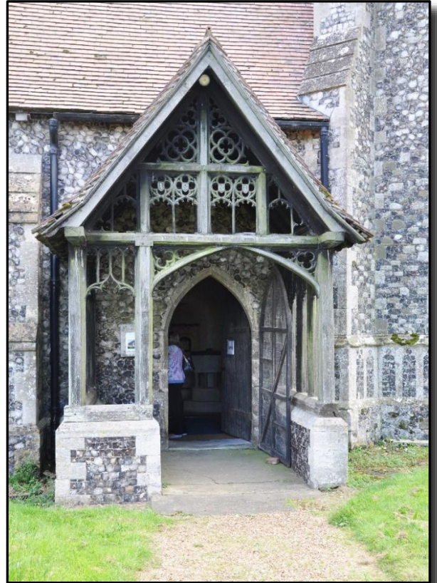
The C19 north porch has a gabled timber frame, perpendicular-style tracery and a flint and stone base.
