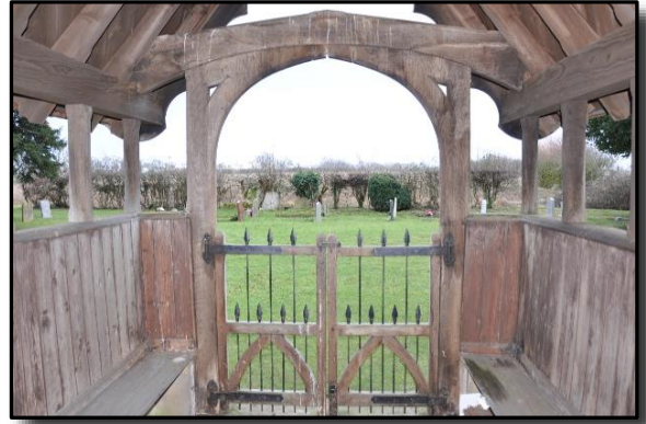
Entrance to the church is via the wicket gate of the south porch just inside which there is a notice telling us that . . .
