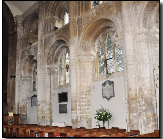
Note the massive Norman pillars and rounded arches. There were of course originally spaces between the pillars which led into a lateral aisle but in C17 the aisles were removed, the lower part of the spaces filled in and windows inserted in the upper parts.
