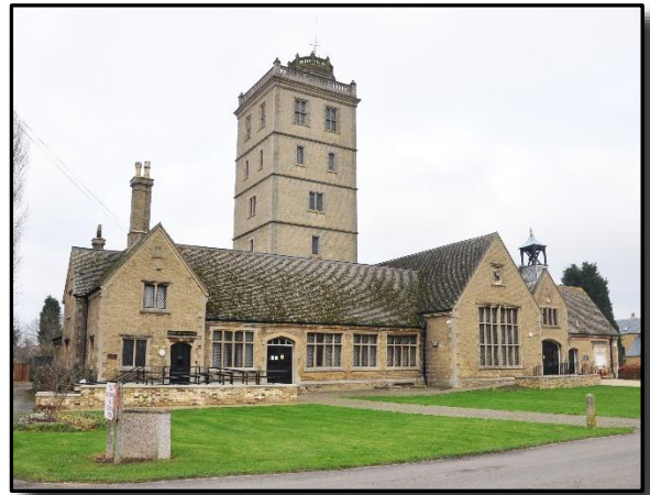
Thorney Heritage Museum is located just 400 metres north of the abbey, in the Tankyard at Bedford Hall in Station Road (PE6 0QE). Its location is marked in green on the map at the beginning of this article.
