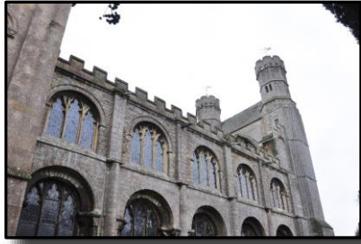
The C12 north wall mirrors the south. Before the removal of the aisles, this was an inner wall. The oolitic limestone of which much of the original part of the church is built, came from quarries at Barnack which were owned by Peterborough Cathedral. This is discussed a little further in Correspondence at the end of this newsletter.
