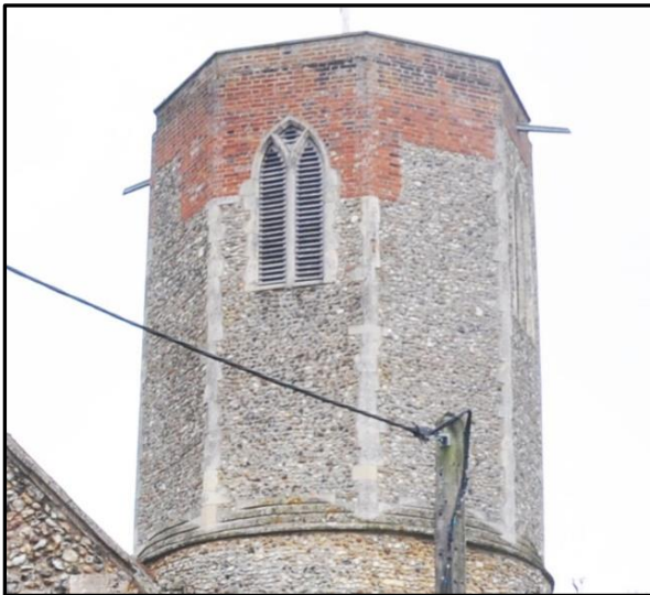
Some of the upper-works have been repaired with red brick.
