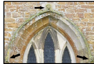
The Statement points out that “the West end has a triple lancet window with a hood mould having two ugly female heads as hood stops.”
