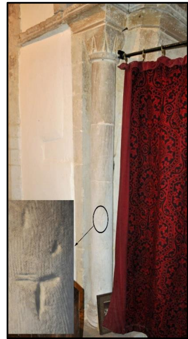
. . . and from this we read that right at the back of the church at the south east corner of the tower, stands a Norman column with a scalloped capital.
