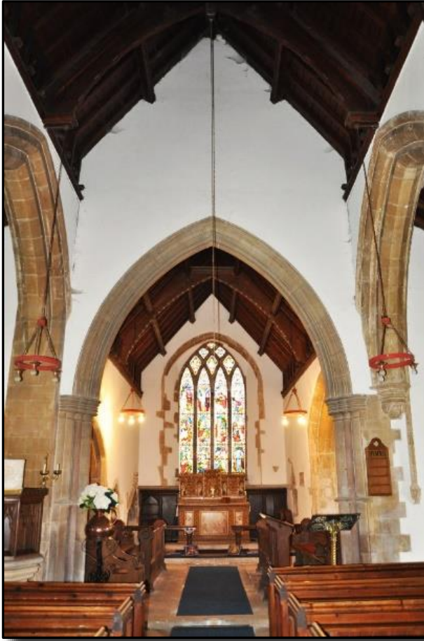
The steep pitch to the roof and the fact that its apex is so high above the apex of the chancel arch, is further evidence of the earlier presence of a clerestory.
