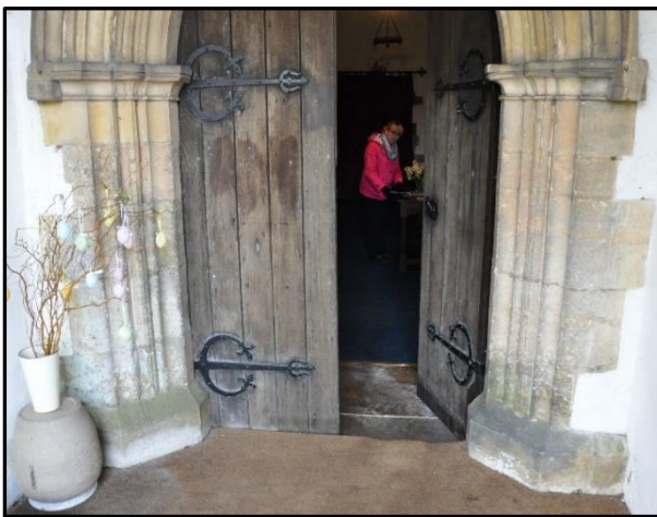
It is C13 and is described as having a wave-moulded outer arch with engaged shafted reveals.
