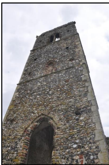
The west face of the tower.
