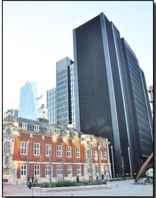
The latest version of his school now resides on the opposite side of Aldgate Square. Although somewhat dwarfed by its massive neighbours it looks quite comfortable here.
