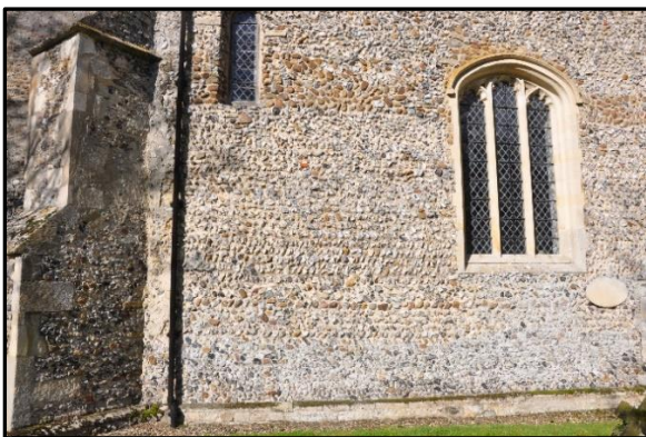
The striations and herring-bone work of this wall are an indication that it was built in several phases.
