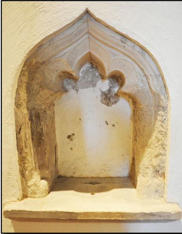
Piscina topped with an ogee arch dating from late C14 and found in the south wall of the south transept.
