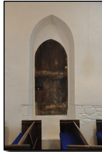
The sealed south door dates from c. 1210 and is set rather too high in the wall to be of practical use today. Until C19 all the previous floors of this church sloped in accordance with the angle of the ground on which the church was built but in c.1875 'a great levelling operation was undertaken' - hence the discrepancy between this door and the floor.
