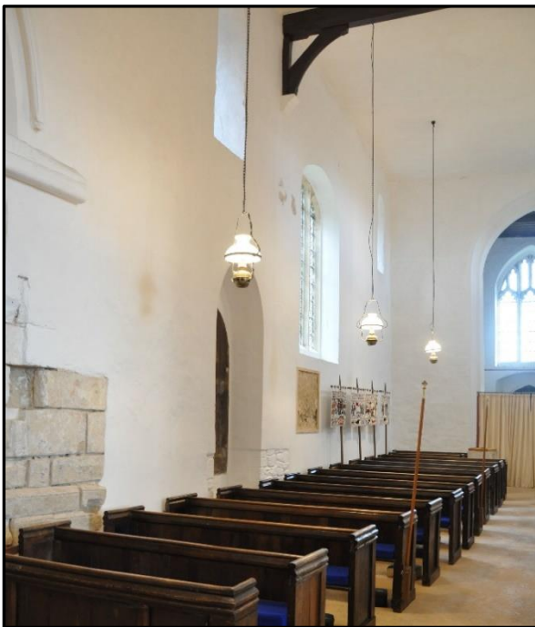
Looking obliquely to the southwest part of the nave we find the sealed up south door that we saw from outside. We also see two of the six original high Saxon windows with their wide splays. At the far western end of the picture the font is just visible.
