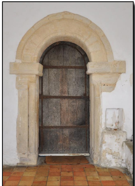
When one first sets eyes on the massively-built main doorway and its door it is immediately clear that one is looking at something special. The door, it is to be noted, is set in line with the inner wall of the church rather than resting centrally on a rebate. This is typical of doorway construction of the immediate post-conquest period.
