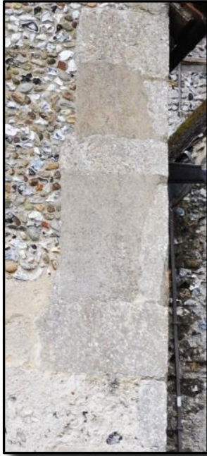
These represent classical 'long-and-short work' found in late Saxon stone buildings.
