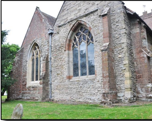
The west end comprises two gabled walls in which both window spaces have been filled with C14-style windows of C19 construction.
