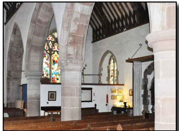
Separating the nave from the north aisle are three pointed archways supported by C14 pillars of irregular pattern - two of which are round in section and the middle one is octagonal.
