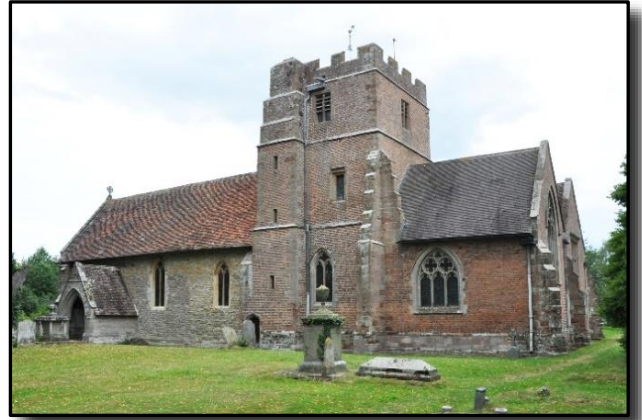
The chancel and tower date from 1674 and are constructed in red brick with red stone dressings which British History Online describes as being an ‘interesting example of Caroline Gothic.’ In the southwest corner of the tower there is a stairway.
