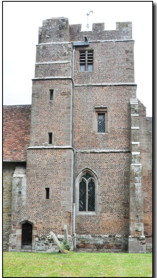
Traditionally, towers in the middle of a church have often been a problem because due to their height and hence their weight they tend to collapse and destabilise the rest of the building. This one seems to be successful in its role. The spiral
