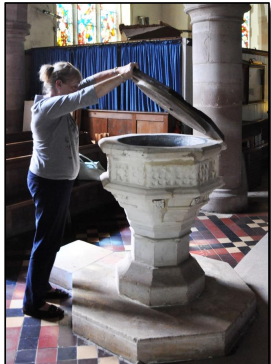
. . . here we can see that on three sides the lower moulding has been removed.
