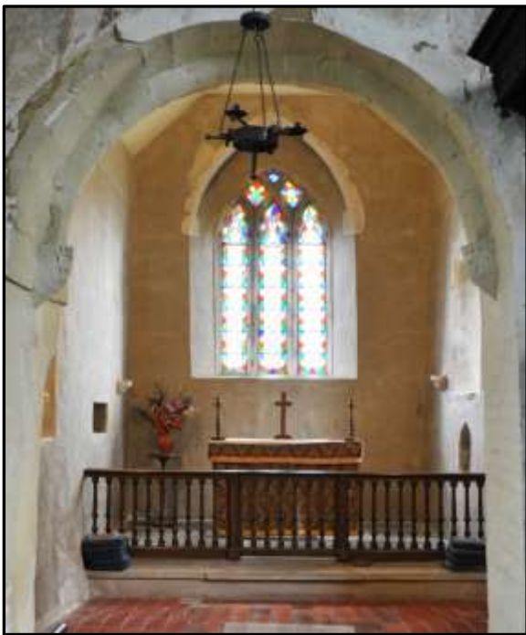
This view of the underside (the soffit) of the chancel arch shows the single Norman soffit roll with end stops.
