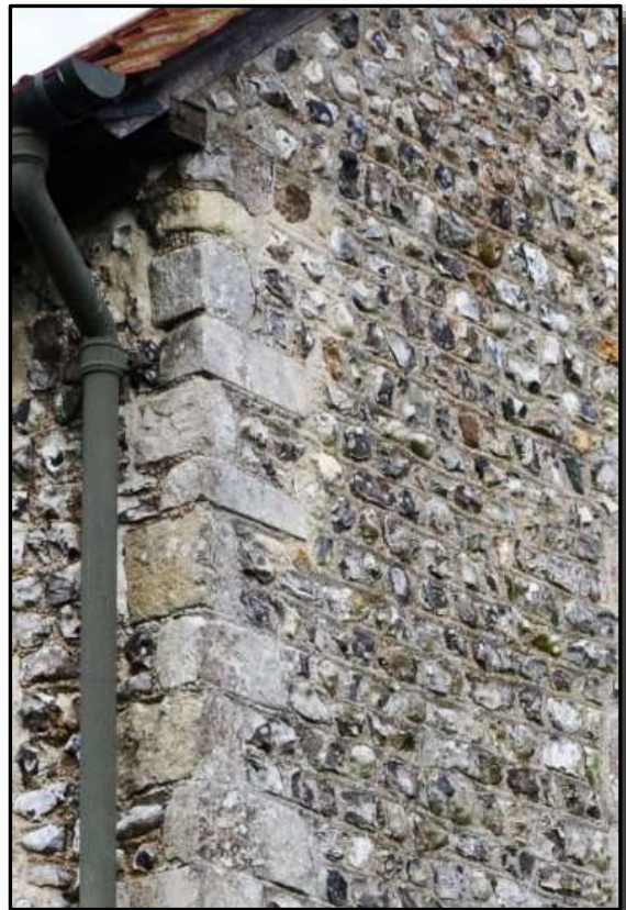
None of them are laid in the 'long and short' configuration favoured by early Saxons.
