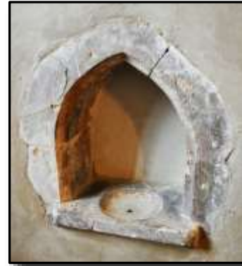
On the south wall of the sanctuary is a simple but attractive C15 piscina and, if you look again at the picture of the chancel, on the north side is an aumbry i.e. a storage niche in the wall. Unusually this one has no doors.
