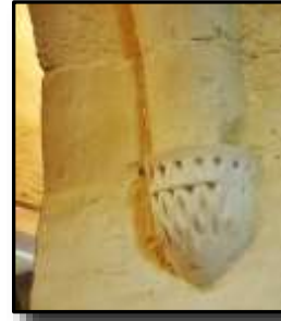
Who can get excited about a soffit roll end-stop? Well clearly I can when they are as old as this one (late Saxon).
