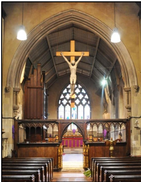
7. The Rood Screen is the oldest to be found in a parish church in Kent. It was constructed in 1370 and originally had solid oak doors and was topped by a rood (crucifix).
