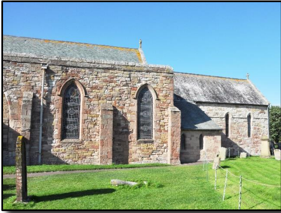
The south aisle of the nave, with its (rather-too-wide-to-be-original) Early English style Gothic windows, dates from 1304 when it was founded as a Chantry Chapel by William de Goswick. To the east of this is the newer C14 chancel built around the smaller original apsidal chancel.
