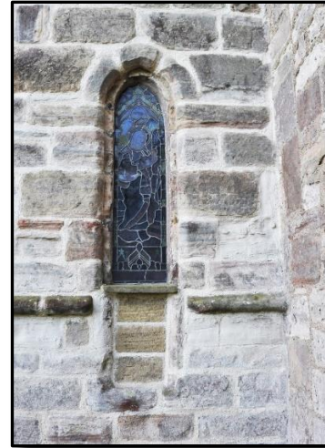
The lower part would have been blocked some time after 1350 but have been open at eye level when it was first installed which would have been soon after 1230 ...
