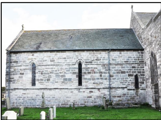
More lancet windows in the C13 north wall of the chancel. and here we have a classic example of a Low Side Window of the type mentioned previously in relation to the Priory Church. Note
